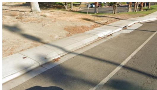
Figure 4. The existing vehicle access driveway on the west side of the intersection will be reconstructed to provide for a wide ADA pedestrian ramp to accommodate bicycle and pedestrian traffic.
