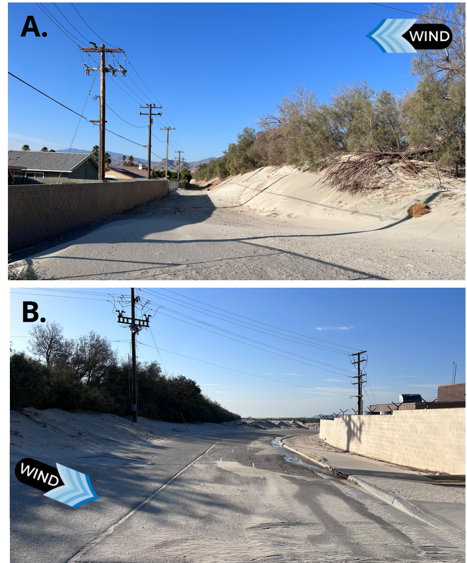
Image 9: Example of influence of bluff objects on sand accumulations
