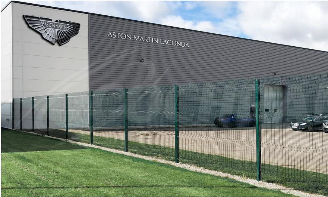
Proposed Fence Design – Height = 8 ft - No cut, no climb with 3 ft shutter barrier.
